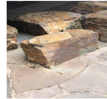
Existing Slate Paving
