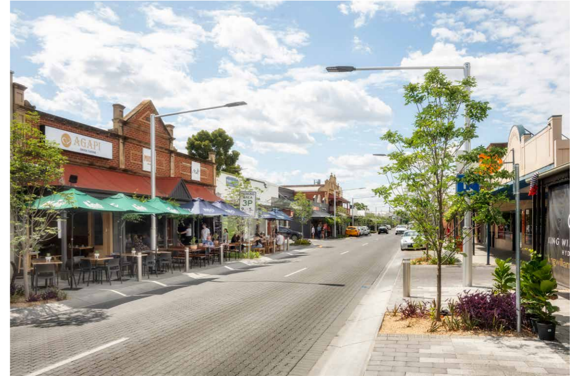
Lane narrowing assists in reducing speeds by reducing the right of way and making drivers more wary of traffic and adjacent road users.
