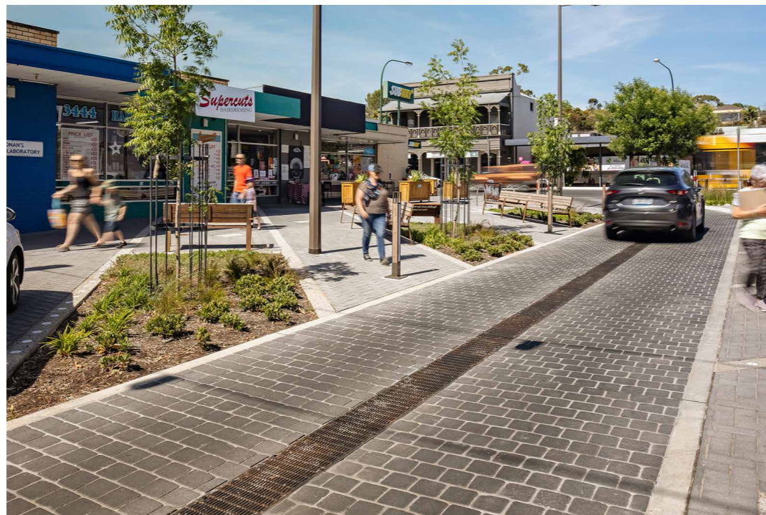
Pavement materials add visual interest, highlight crossing areas indicate a change in conditions to drivers and pedestrians.
