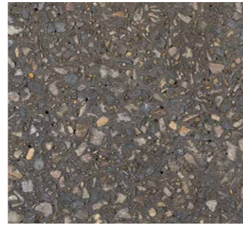
Exposed aggregate concrete (roadway)
