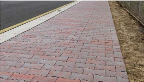
Permeable Paved Footpath
