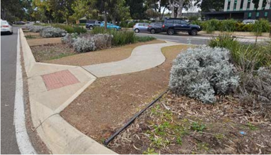
Kerb ramp crossing
